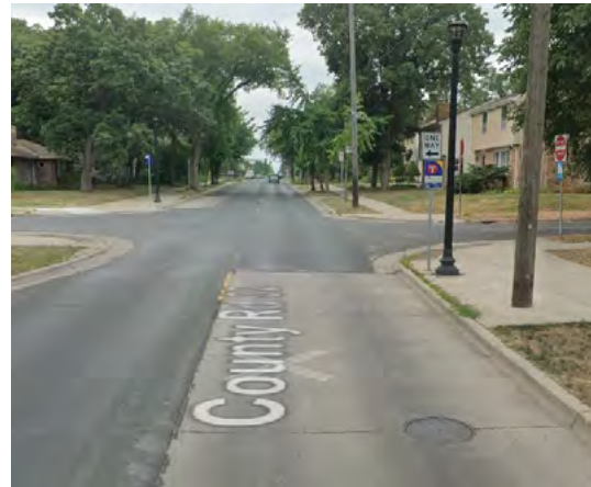
In-lane stop without a median. Penn Ave. S. at W. 53rd St., Minneapolis
