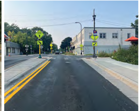
In-lane stop with short center median. Johnson St. NE at 22nd Ave. NE, Minneapolis
