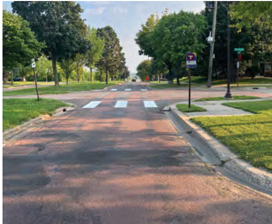
In-lane stop with block length median and pull-out parking bays. Stinson Parkway at 19th Ave. NE, Minneapolis
