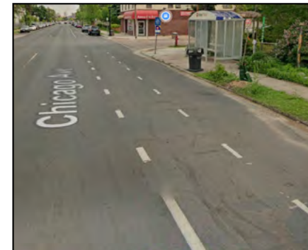
Figure 48 Example of a bus bike mixing zone on Chicago Ave. S. at E. 32nd St.
