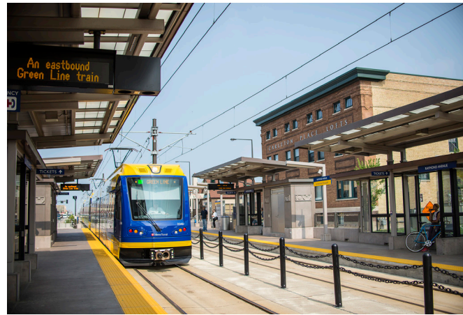
Raymond Avenue Station on the METRO Green Line
