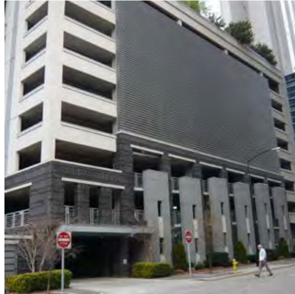
Figure 4.20 Integrate new structured parking into the development. While this structure shows appropriate screening, it is not wrapped by active uses as the design guidelines instruct.
