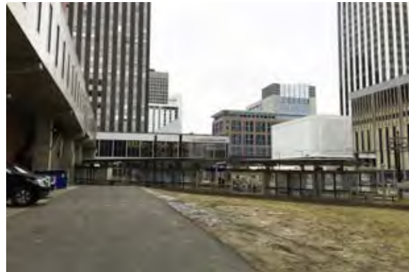
Figure 5.11 Maintain the service drive on the east side of the Saint Paul Athletic Club (shown above).
