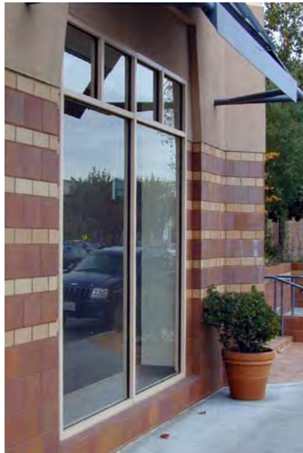
Figure 4.12 Employ materials at the ground level to withstand on-going contact with the public without compromising the appearance.
