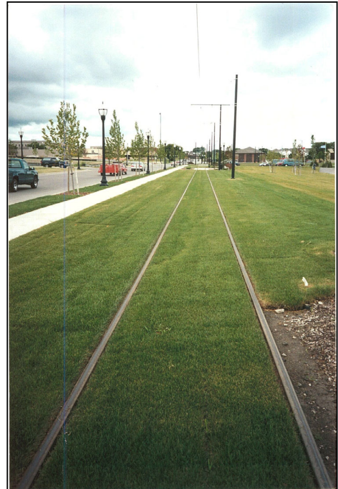
The Kenosha, Wisconsin line has grass between its tracks, beautifying the area, and reducing noise. Electric power, continuous-welded tracks, and "resilient" wheels also substantially reduce sound levels.
