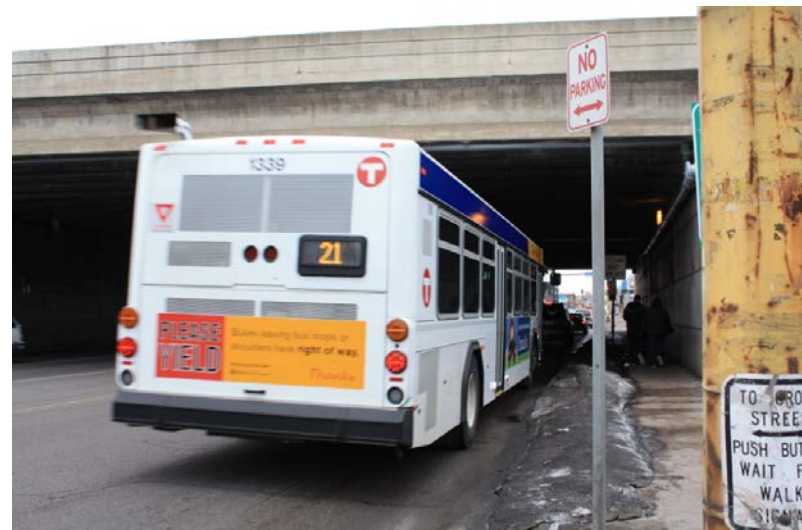
Existing Lake Street bridge conditions
