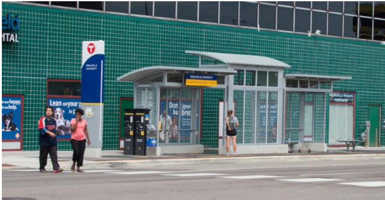
Figure 18: Large shelter on the A Line, Snelling & University station
