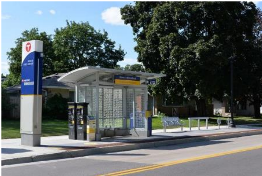
Figure 8: Arterial BRT shelter
