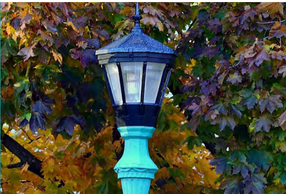
Light fixtures are typically the lantern-style shown here with high hand holes to prevent wire theft.
