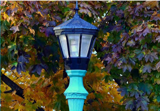
Light fixtures are typically the lantern-style shown here with high hand holes to prevent wire theft.
