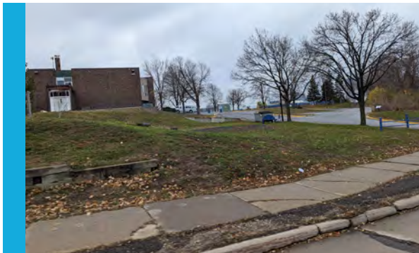
Sidewalk on Jackson St with evidence of deterioration due to water and ice.
