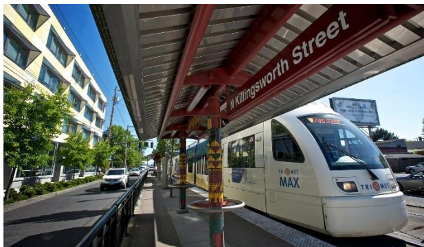
Portland Yellow Line LRT
