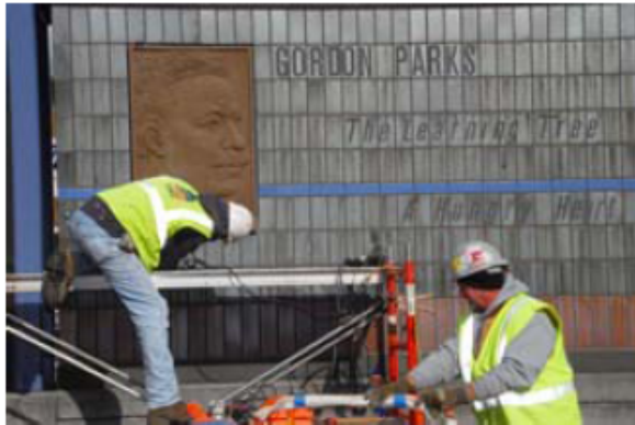
Crews install a terra cotta panel with a likeness of Gordon Parks as part of the Victoria Street Station's "Faces of Rondo" artwork. (Photo courtesy of Metropolitan Council)
