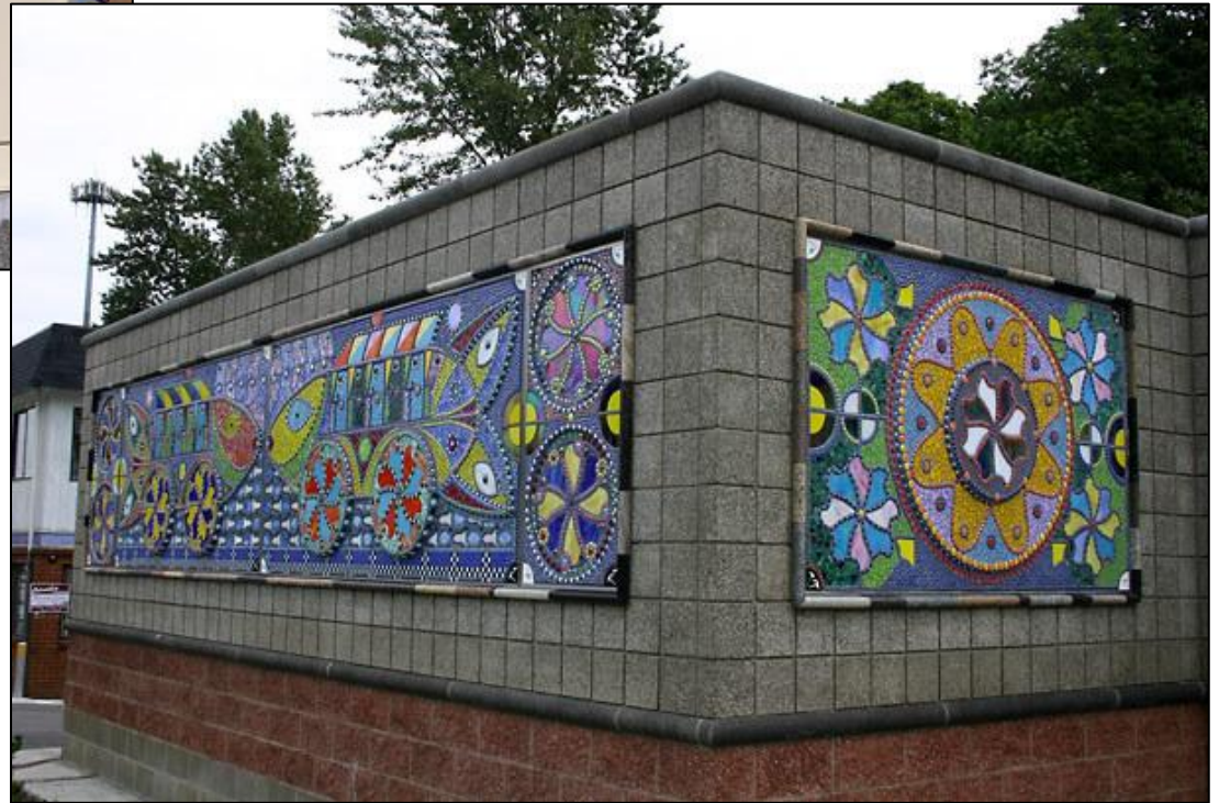
Traction Power Substation Sound Transit Central Link LRT, Flores, Fishmobile and Pinwheel, Mauricio Robalino, artist
