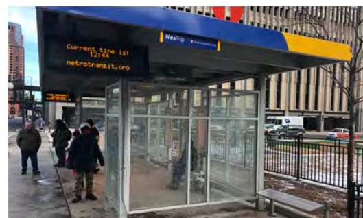
Stop Reference: 2015 Improvements
