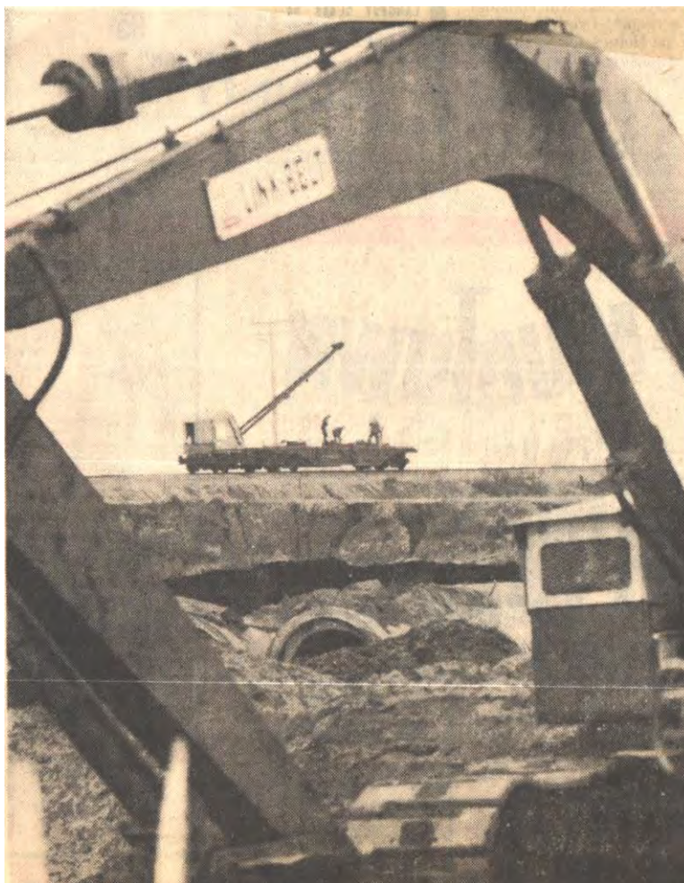
Figure 8. Bridge 62529 under construction in November 1974. This photograph shows the track on the existing berm, which will be cut out to allow the construction of the bridge and highway. 658
