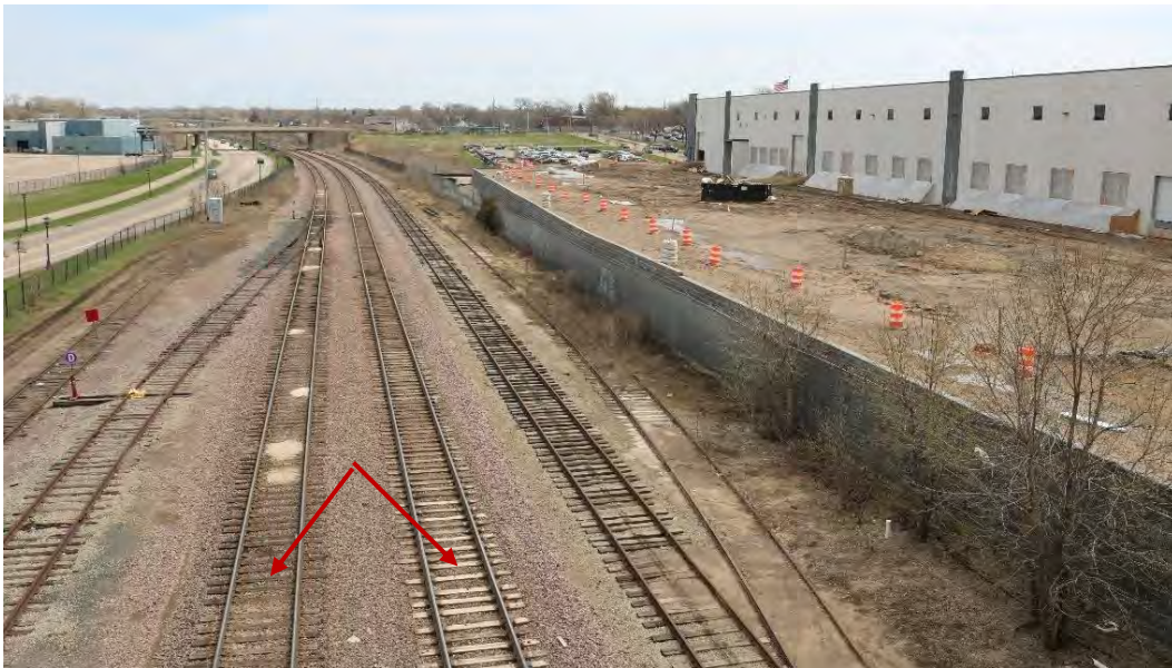
Figure 9. Image of the corridor from the Arcade Street Bridge, view facing east. Note that that the additional trackage is reduced to three tracks east of Arcade Street (red arrows indicate the mainlines). Also note the presence of former sidings. The parcel to the south (right) of the corridor was historically the 3M campus and is currently being redeveloped.
