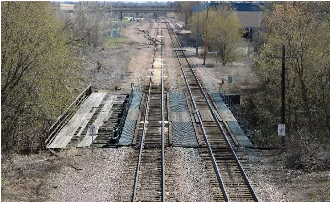
Figure 6. Image of the corridor from the Payne Avenue Bridge, looking east, showing the deck girder bridge (RA-SPC-11130) that carries the corridor over the Phalen Creek valley and the historic alignment of the LS&M. Beyond the bridge, note the addition of sidings to the double track.
