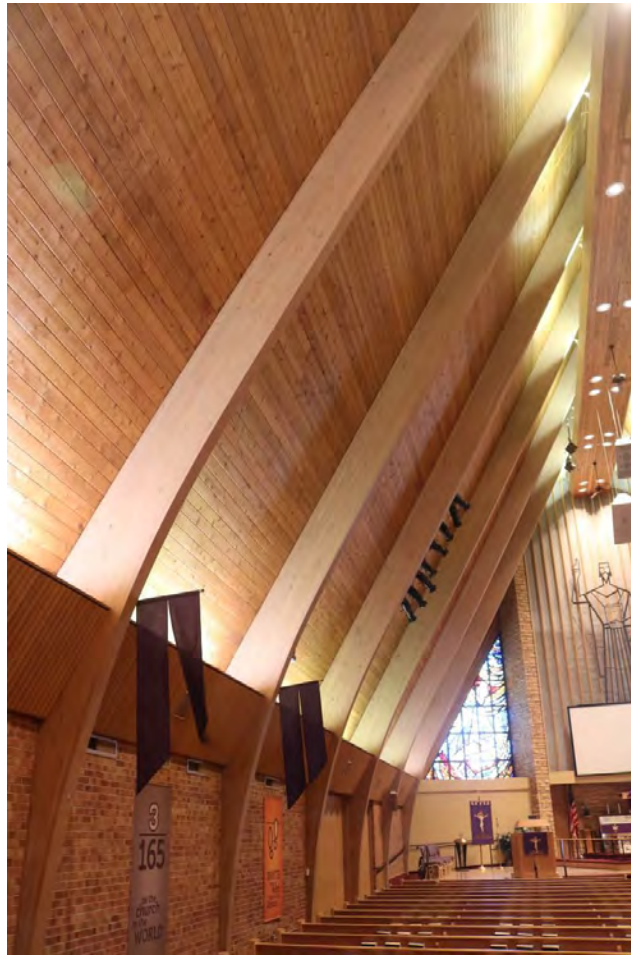
Figure 20. Image showing beadboard panels between the laminated trusses at the top of the brick knee walls.
