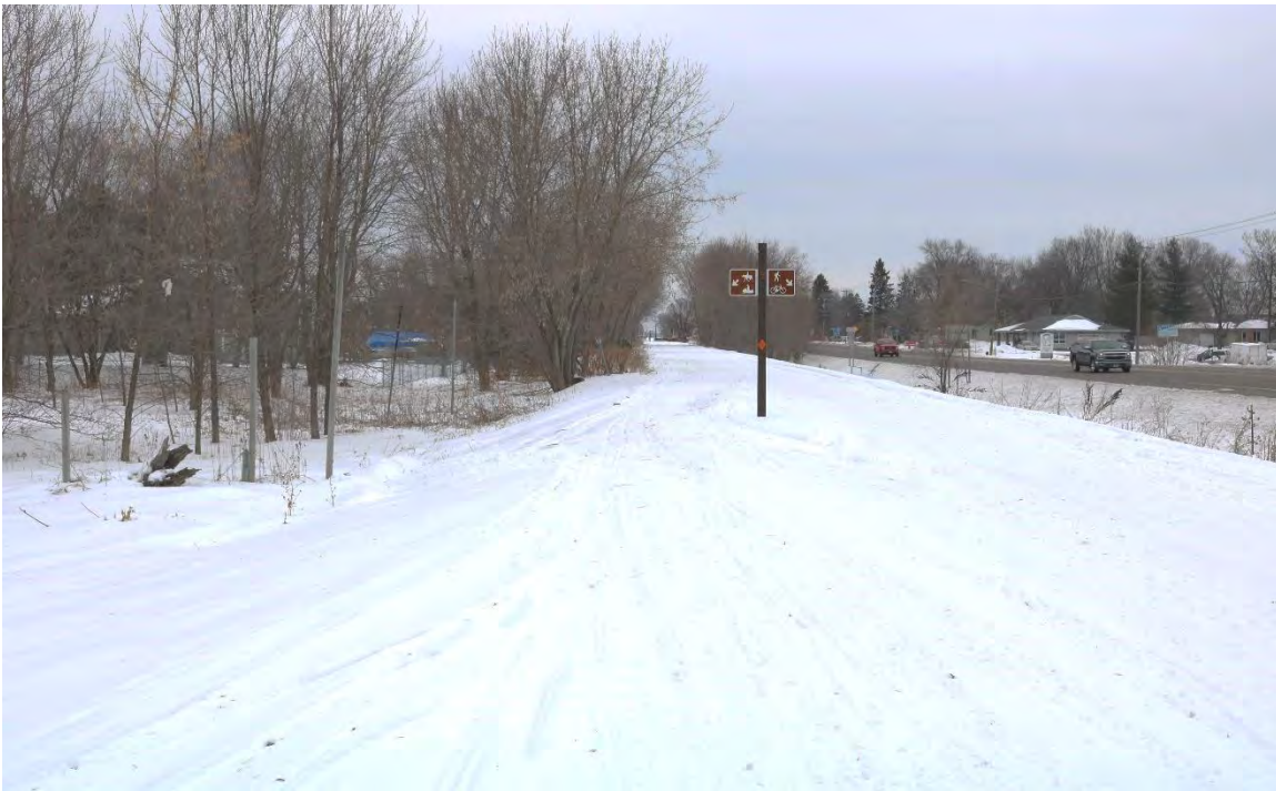
Figure 16. Image of the LS&M railroad roadway at 140 th Street, view facing north, showing the presence of the raised railroad roadbed and ditches. The roadbed is currently carries the Hardwood Creek Regional Trail. Trail signs are located within the railroad roadbed.
