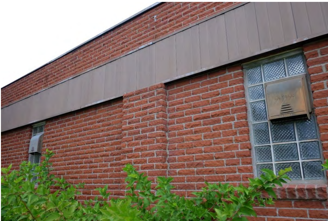
Figure 10. Window openings in 1964 building with diamond patterned/textured glass block and metal exhaust fans. One of the two pilasters on the 1964 elevation is also showing. View facing east.
