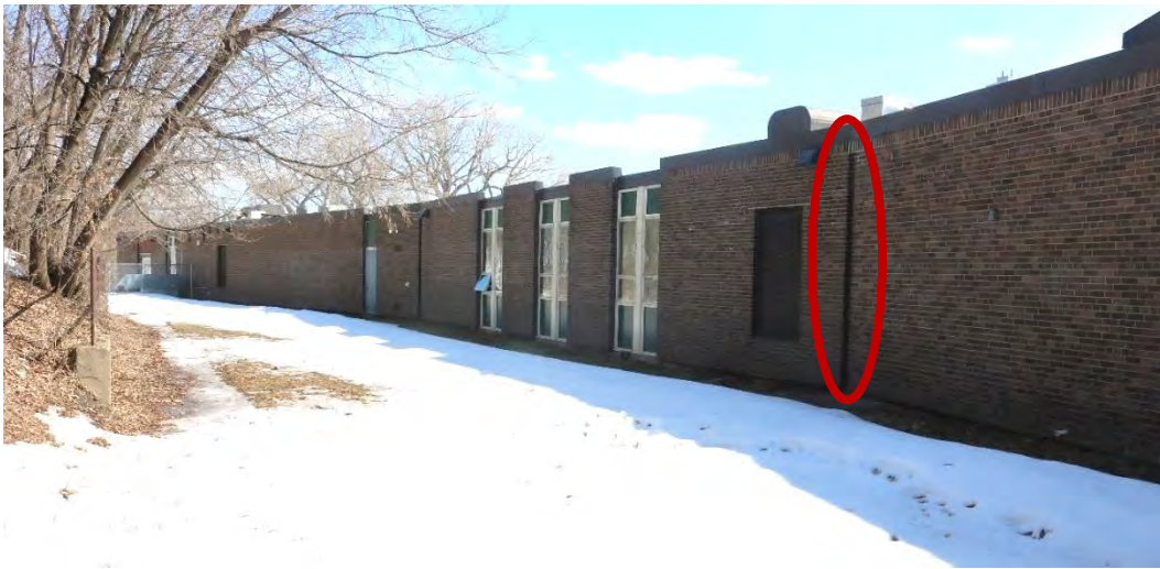
Figure 12. Rear (north) elevation east of the gymnasium addition with full-height paired window bays and secondary entrances, looking southeast. Note the narrow vertical recessed bay (encircled in red) that denotes the different blocks of the building.
