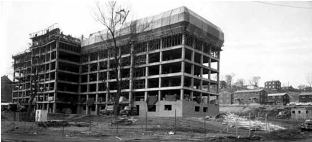
Figure 21. Construction of the high-rise in April 1958 showing its reinforced-concrete structural system. 19
