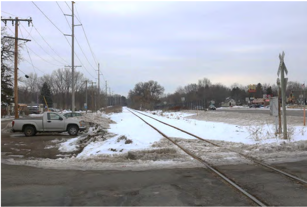
Figure 4. Image of the LS&M railroad roadway showing the non-automated crossing at 8 th Street in White Bear Lake, view facing north. Note the presence of signage at the crossing.
