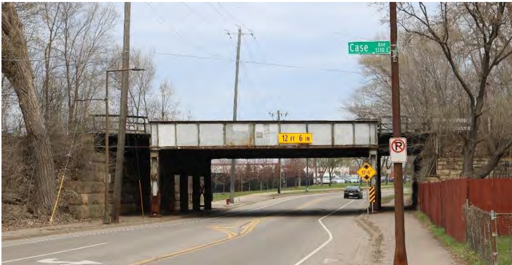
Figure 13. Image of the corridor as it crosses above Johnson Parkway on the 1906 steel-through-girder bridge, looking north.
