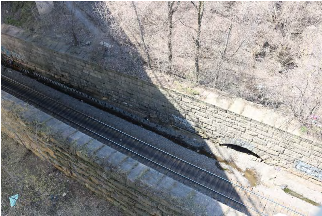
Figure 11. Partially visible arch, likely part of one of the east-west culverts built into the retaining wall between the northern portal of Westminster Tunnel and the southern portal of the western, 1885 North End Tunnel.
