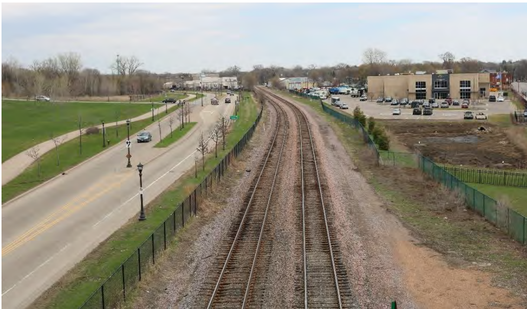
Figure 11. Image of the corridor from the Earl Street Bridge, looking east. Note that the triple track is reduced to a double track at Earl Street.
