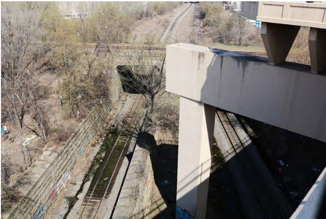
Figure 9. Looking north from the Phalen Boulevard Bridge showing the western, 1885 North End Tunnel and the retaining walls (one on each side of the track) that extend from the north portal of the Westminster Tunnel to the south portal of the 1885 North End Tunnel. The bridge superstructure in the foreground is part of the 2004 Phalen Boulevard Bridge.
