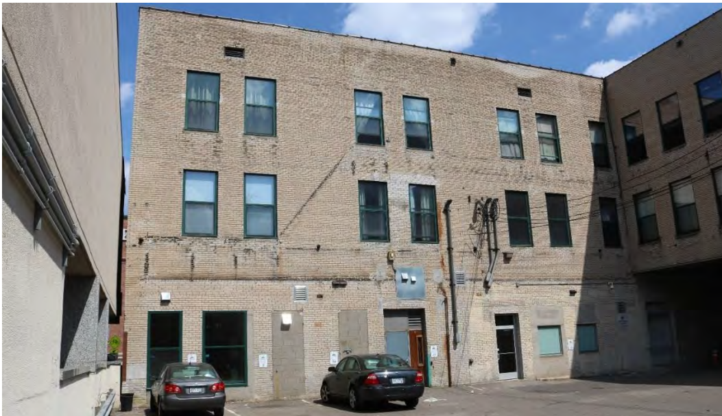
Figure 9. Southwest-facing interior elevation, view facing east. Window and door openings on the first story have been altered, and portions of the brick have been infilled with concrete block.
