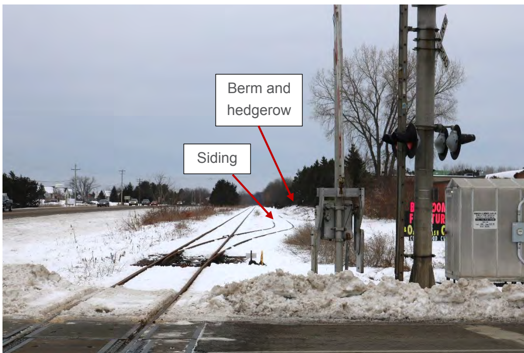
Figure 12. Image of the LS&M railroad roadway at 130 th Street, view facing south. Note the automated crossing signal and moveable arm at right and the siding trackage at center. The siding is separated from the light industrial properties to the west (right) by a berm and hedgerow of pine trees.
