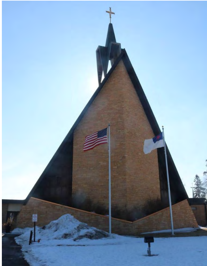
Figure 6. Front gable of the 1963 A-frame sanctuary, view facing east. Note the three parts that make up the prow-like front gable: the triangular central stone section, two multi-light glass panels, and a triangular stone planter with metal coping.
