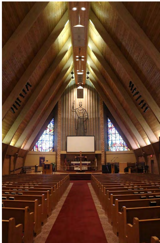
Figure 18. 1963 A-frame sanctuary, view facing west. Note how the curved laminated trusses extend from the peak of the ceiling to the floor. Also note the catwalk that spans the length of the sanctuary. Access to the catwalk is located on the west wall behind the central panel of the altar area platform.
