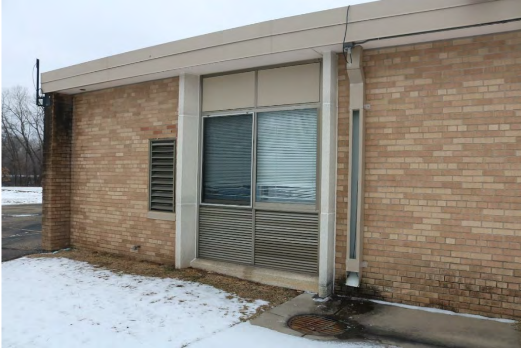
Figure 3. Typical window bay composition with full-height pilasters and an adjacent ventilation grate, view looking northwest.
