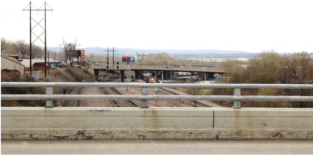
Figure 2. Looking southeast from the Lafayette Road Bridge. Note how the tracks are at similar grades before entering Westminster Junction and how the rail corridor sits below the surrounding landscape, represented by the bridges that run at grade.
