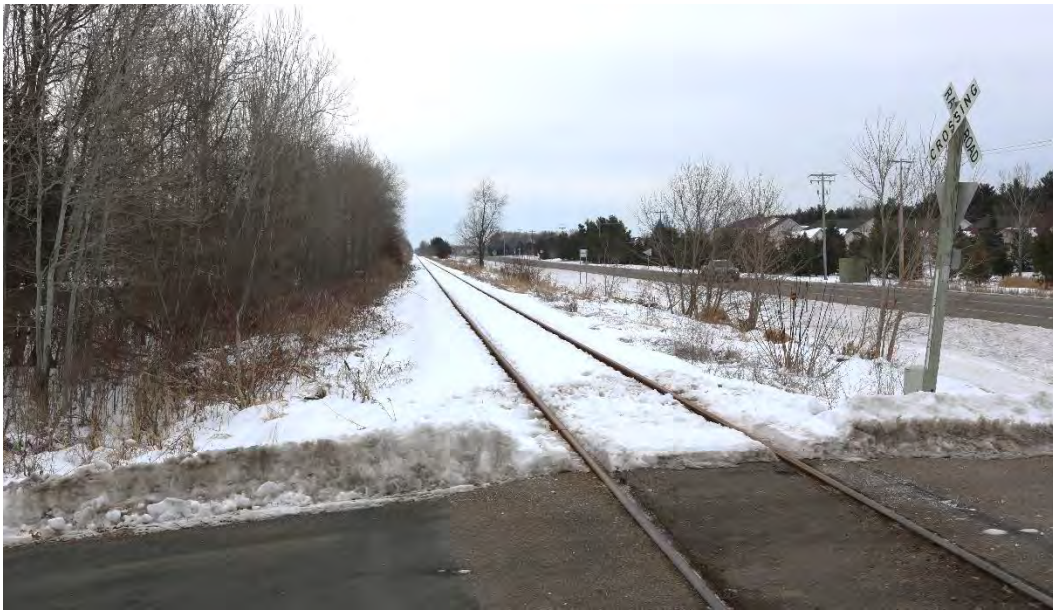
Figure 11. Image of the LS&M railroad roadway at 125 th Street, view facing north, showing the non-automated crossing at that intersection.
