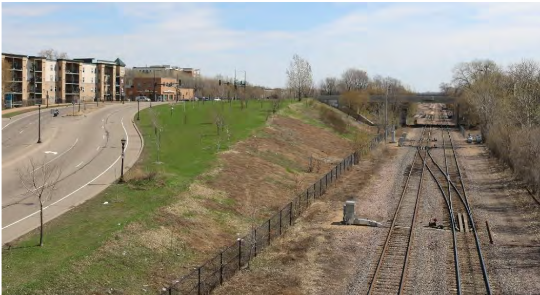
Figure 5. Image of the corridor from the Edgerton Street Bridge, looking east. The fill embankment to the north (left) of the corridor was constructed as part of the Phalen Boulevard project, connecting Phalen Boulevard and Payne Avenue. The bridge visible in this image carries Payne Avenue over the corridor.
