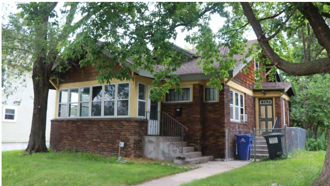
Figure 76. This side-gable bungalow at 780 Capitol Heights (RA-SPC-10153) in Saint Paul was constructed in 1922 and features overhanging eaves with brackets, a partial-width front porch and brick cladding.
