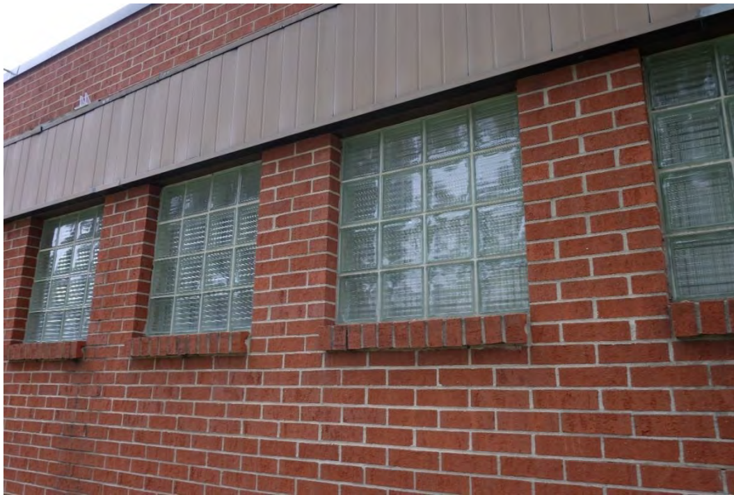
Figure 11. Four of six of the smaller window openings in the ca. 1980 addition with square patterned/textured glass block. View facing east.
