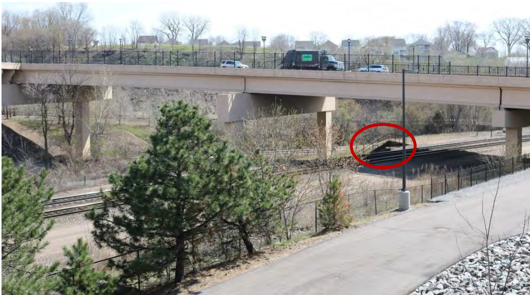
Figure 13. View from west of the junction facing southeast showing the 2004 Phalen Boulevard Bridge crossing the double-track, western leg of the upper wye. A small portion of the north portal of Westminster Tunnel is visible in this image, marked by the red oval.
