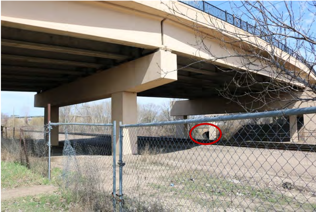
Figure 14. View from west of the junction facing north showing the 2004 Phalen Boulevard Bridge crossing the northern portion of the junction. The double-track, western leg of the upper wye is visible at center and part of the eastern, 1888 North End Tunnel is also visible and marked with a red oval. Note the pairs of concrete piers placed within the junction.
