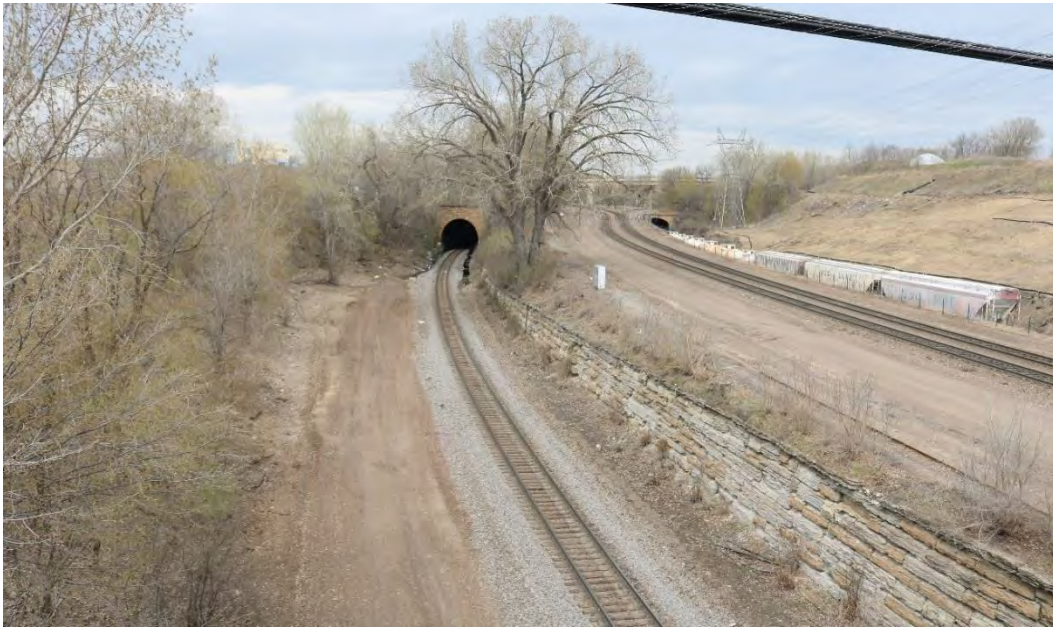
Figure 4. Looking northwest from the Lafayette Street Bridge showing the grade separation at the south end of the junction. The raised center grade (at right) has a double track while the West Side Line (at center) has a single track and a roadbed lower than the center grade. The southern portal of the Westminster Tunnel is visible on the left as are the train cars on the East Side Line on the right. Note the ashlar-stone retaining wall at center.
