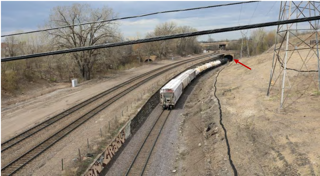
Figure 3. Looking northwest from the Lafayette Road Bridge showing the grade separation at the south end of the junction. The raised center grade (at right) has a double track while the East Side Line (at center) has a single track and a roadbed lower than the center grade. The southern portal of the East Side Line tunnel is visible in the background at the end of the train at center (red arrow). Note the counterfort stone retaining wall.
