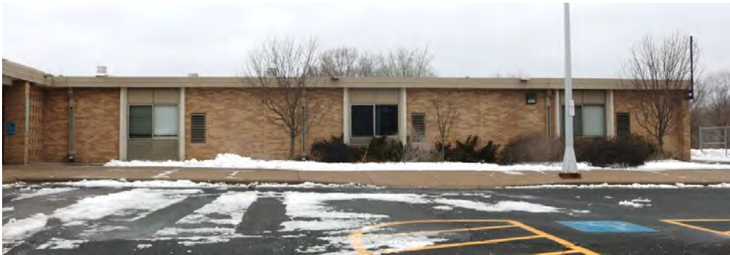
Figure 5. Typical side elevation of a classroom wing with window bay units framed by projecting pilasters and adjacent ventilation grates. This photograph is the east elevation of the north wing, view looking west.
