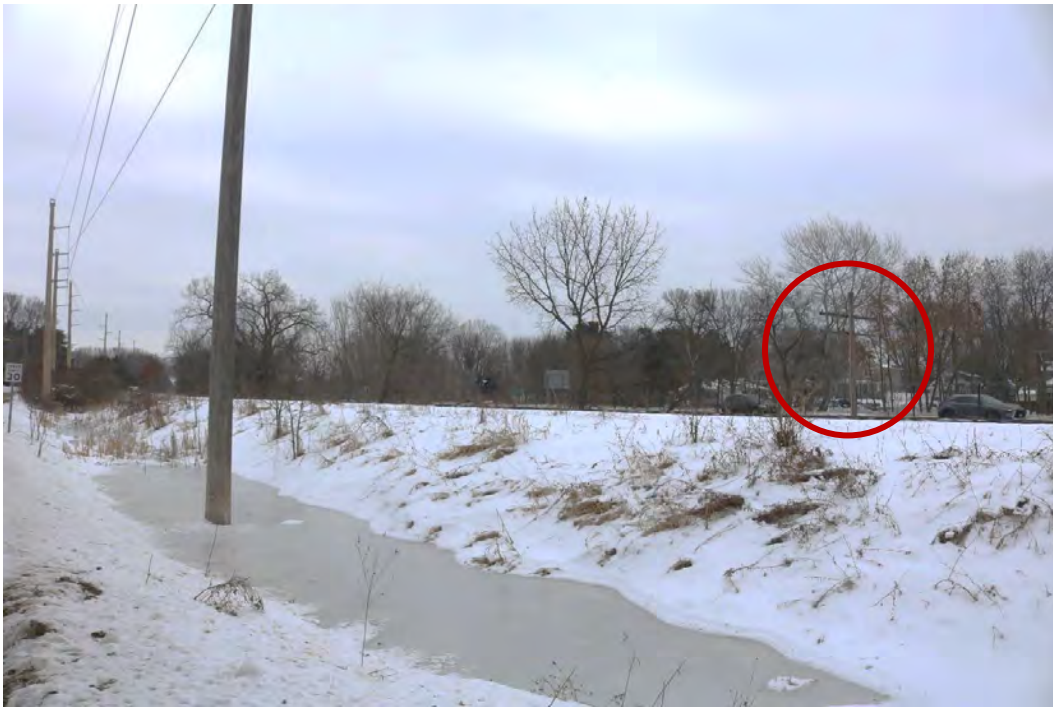
Figure 5. Image of the LS&M railroad roadway , view facing northeast, showing the more pronounced embankment and ditch north of 8 th Street. The embankment carries the active rail line. A wooden utility pole on the east side of railroad roadway is barely visible in this image (circled in red). The vehicle visible near the utility pole is traveling south on TH 61.
