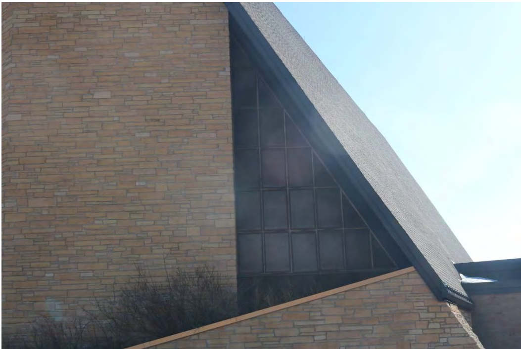
Figure 7. The multi-light glass panel with metal framing that protects the interior stained-glass window. Two panels are found in the front gable, one on either side of the central stone section. View facing east.
