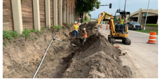
Example of crews placing utility tubes on Orange Line
