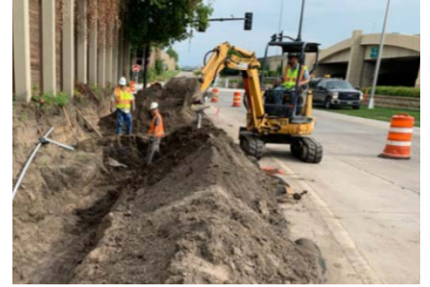
Example of crews placing utility tubes on Orange Line
