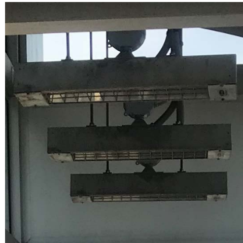
Platform Light & Heaters (A Line Shown)
