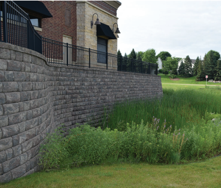
Sheet pile wall with post and picket railing to match existing small block retaining wall
