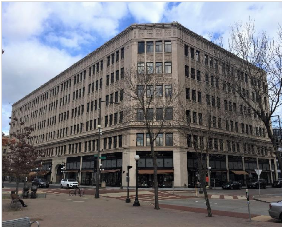
Figure 67. Hamm Building, facing north-northeast
