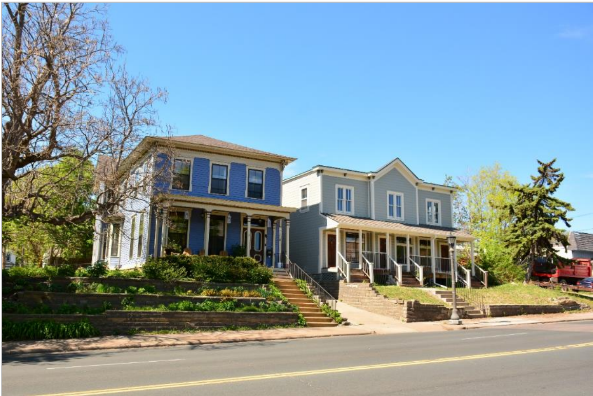
Figure 25. Bell-Weber House (left), facing north-northeast
