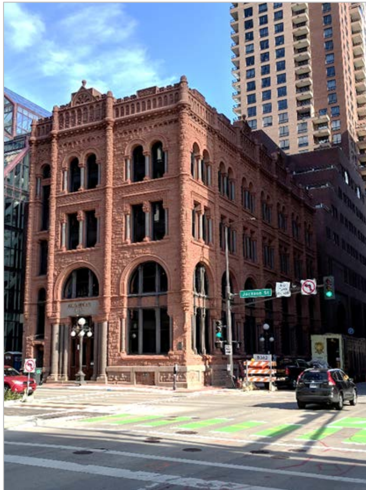
Figure 42. Merchants National Bank, facing northeast
