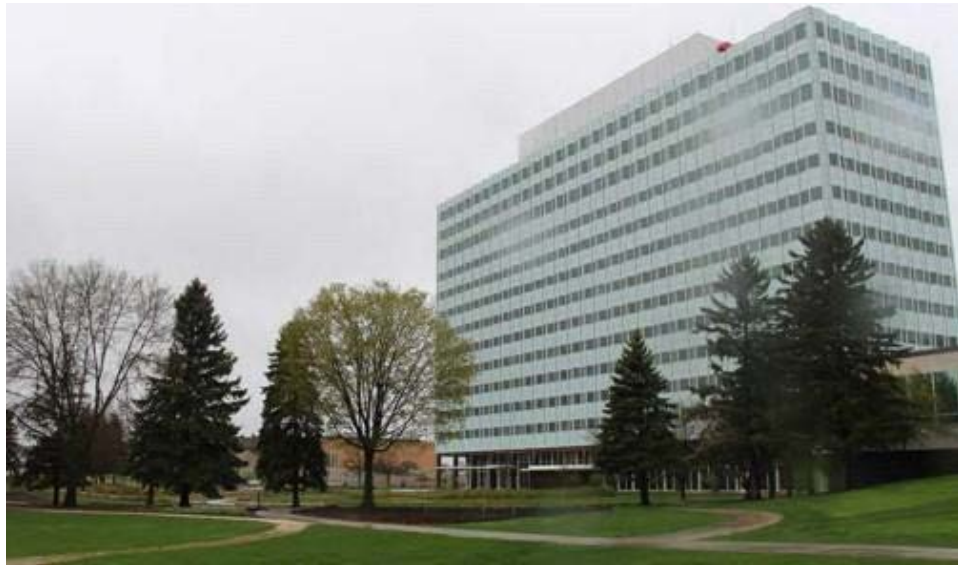
Figure 11. 3M Center, Facing northwest
