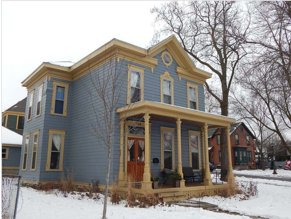
Figure 29. Peter Bott House, facing east
