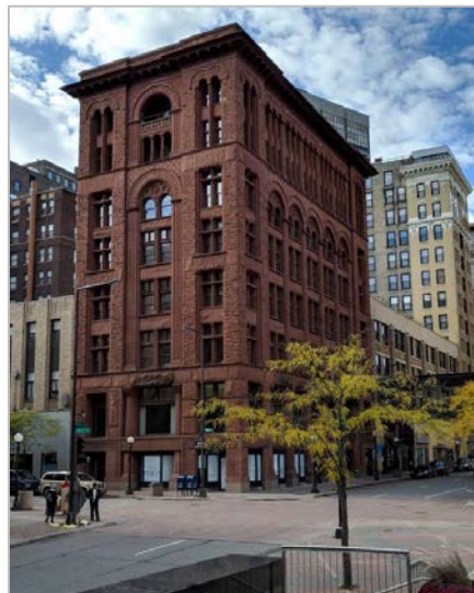
Figure 57. Germania Bank Building, facing southwest
