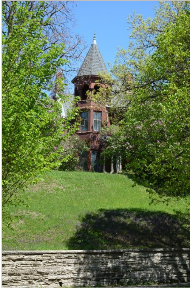
Figure 21. Giesen-Hauser House, facing northeast
