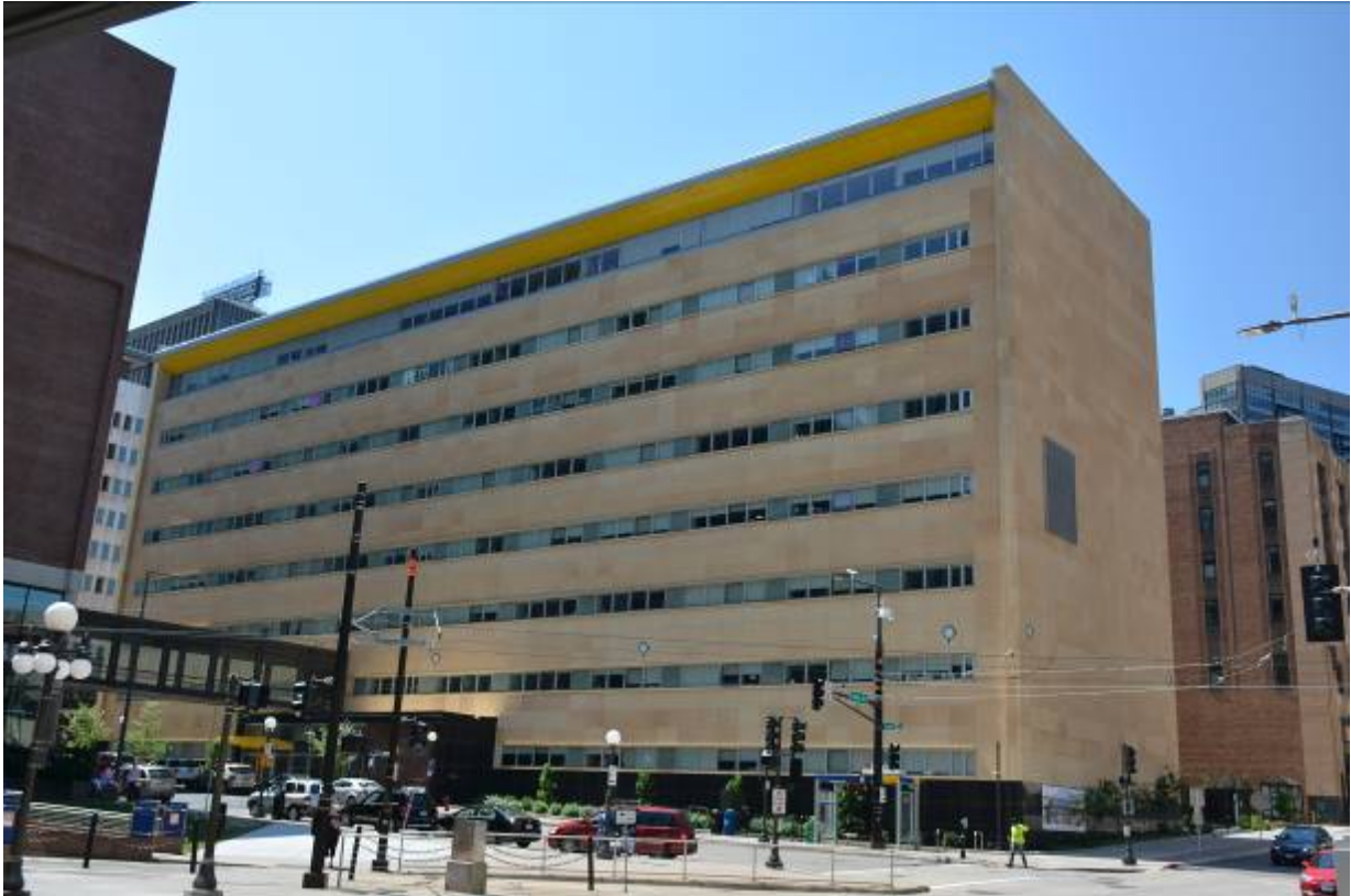
Figure 55. MMLI Building, facing south
