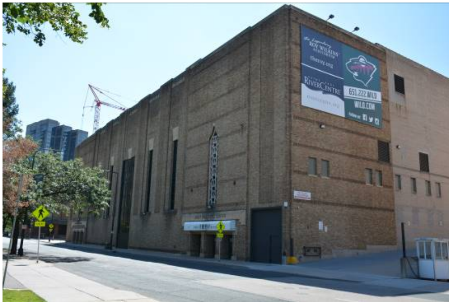
Figure 69. Saint Paul Auditorium Addition, facing east
