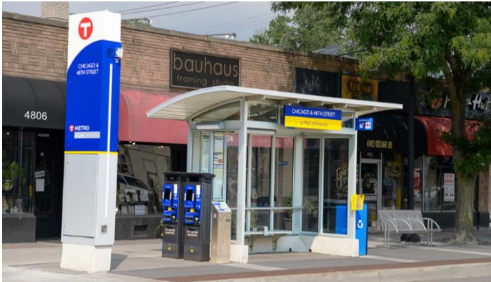
Small shelter 12 feet long, 5 feet wide, and 9 feet high.
