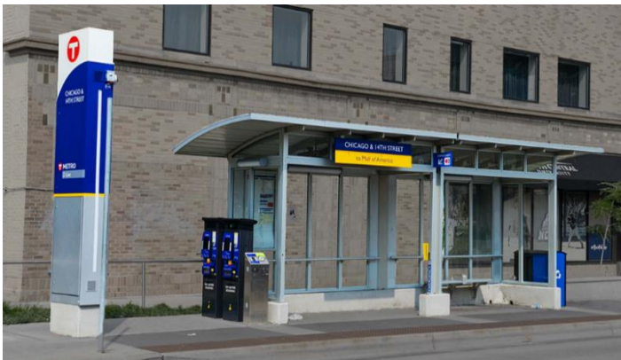
Medium shelter 24 feet long, 5 feet wide, and 9-12 feet high.
