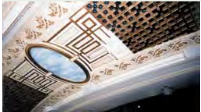
View of under-balcony ceiling during construction. The wide perimeter decorative plaster band is from the original construction. The interlocking central element was recreated using the Tacoma Pantages as a starting point for interpretation. (HGA photo)
