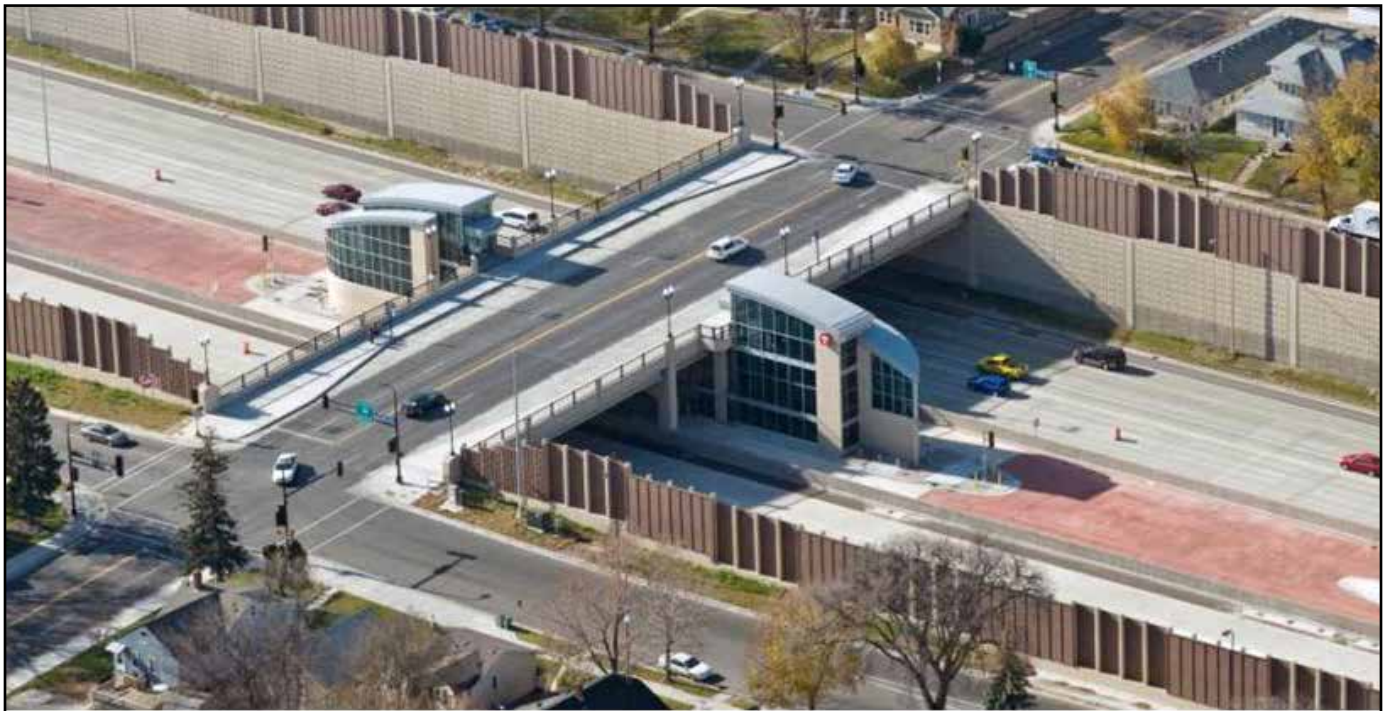
Figure 10. Aerial View of 46th Street Station
