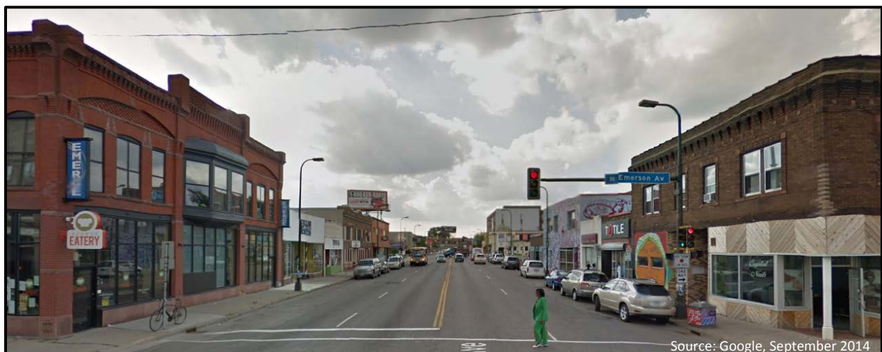
Figure 6: West Broadway Avenue at North Emerson Avenue
