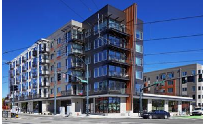
The Prescott, completed in 2014, is a market-rate multifamily development along the corridor.
