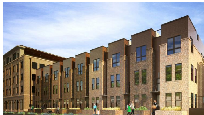
The Wheatley, a luxury, mixed-use, mixed income development under construction at the 25 th and Welton Station.
