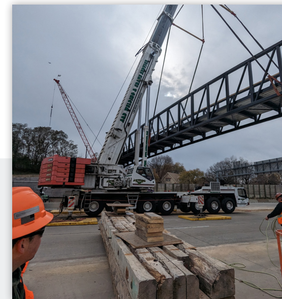
Crews crane the Maple Street pedestrian bridge in place.
