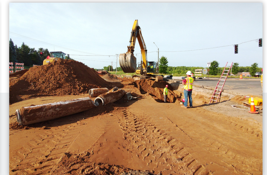
Crews install underground utilities
